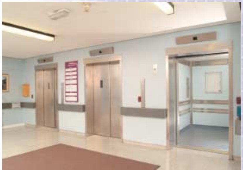
Lifts following completion of modernisation
