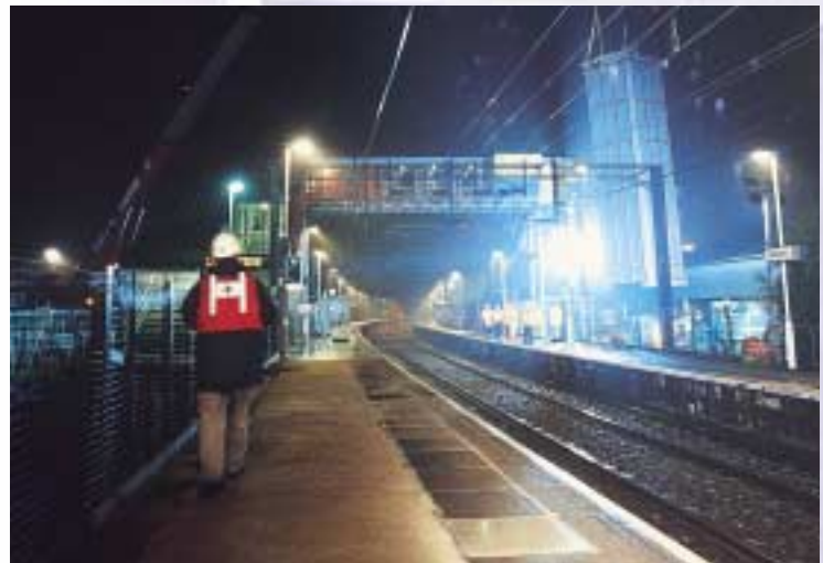
Lift towers fitted in 8 hours
