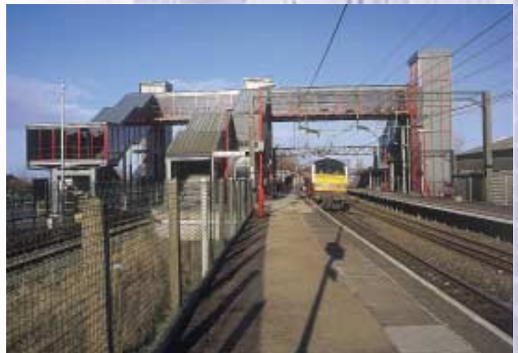
Runcorn Rail Station after, with three new hydraulic lifts
